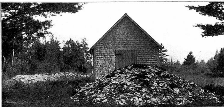
Figure 2.5. Mica grading shack near Cardigan Station, New Hampshire. Sacks of high grade mica are inside the building, lower grade pile of mica in the foreground, and common mica in the background. From Pulsifer (1914:143).
