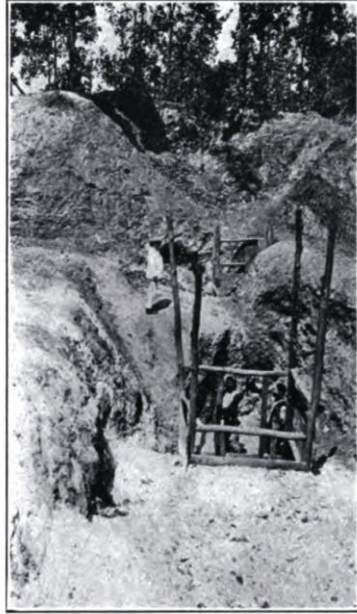
Figure 6.3. Shaft sunk through caved workings, Panya mine, Hazaribagh District, Kodarma, India, ca. 1914. From Dixon (1914:101).
