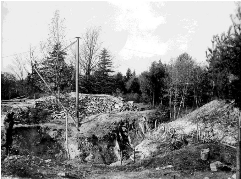
Figure 5.1. Northwestward across the main open cut of the Rhoda Mica mine (also Big mine, Bowers mine, etc.), Alstead, Cheshire County, New Hampshire. Photo before 1923, first worked by James Bowers ca. 1834. Plate 14-A in U.S.G.S. Bulletin 740. 1923. Courtesy U.S. Geological Survey.
