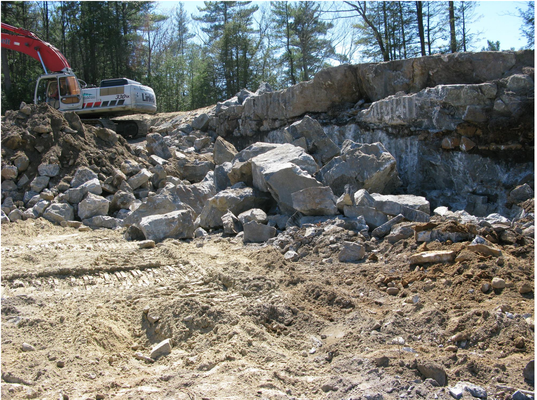
April 2019 Adjacent commercial building parking lot expansion
