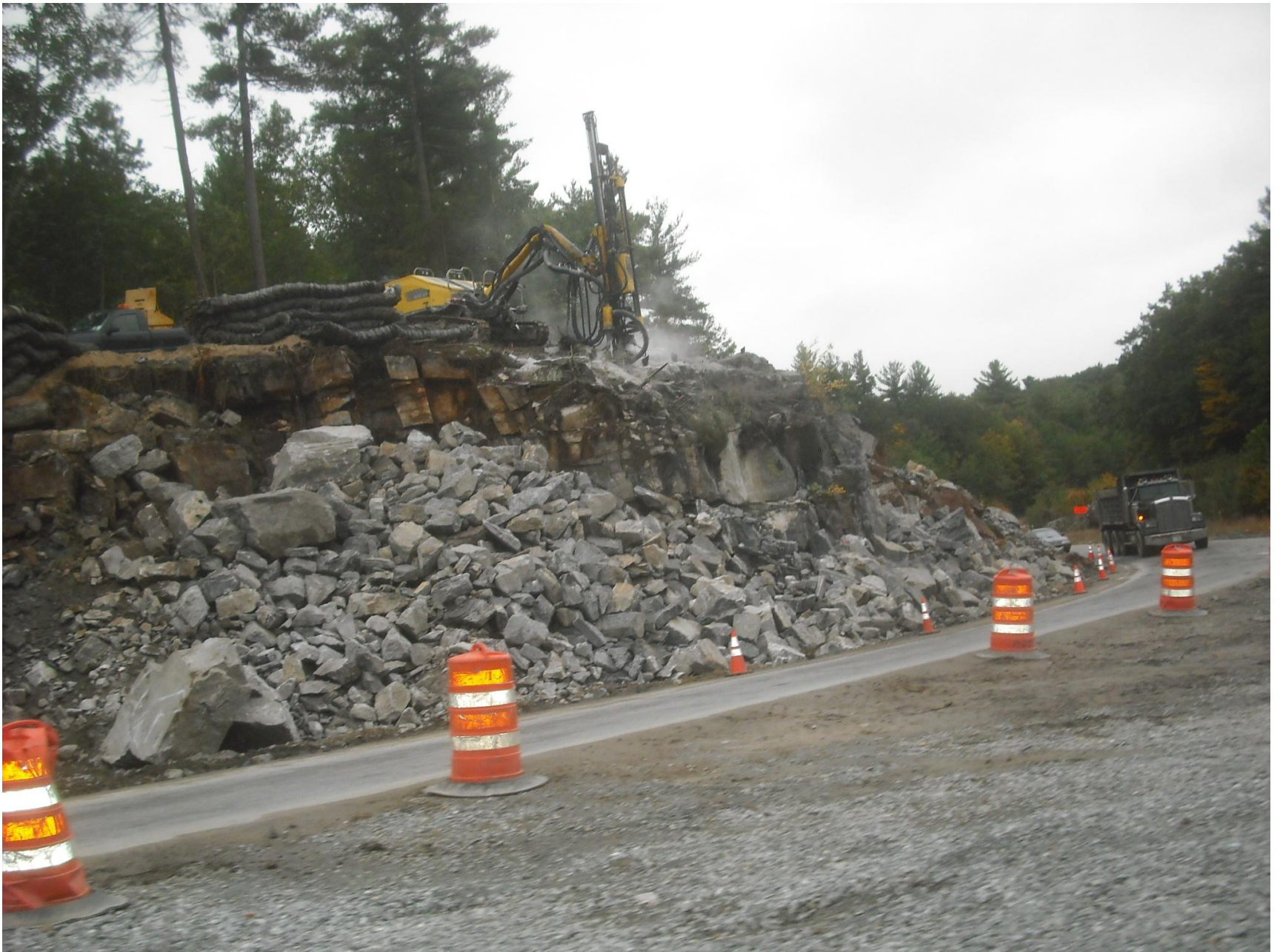
2018 – 2019 Off ramp modification
